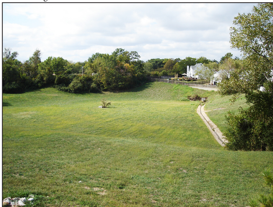
Figure 4. This detention basin near Telegraph Road in Oakville diverts storm runoff into culverts that intersect two caves, including the longest cave in St. Louis County (Stop 4).
